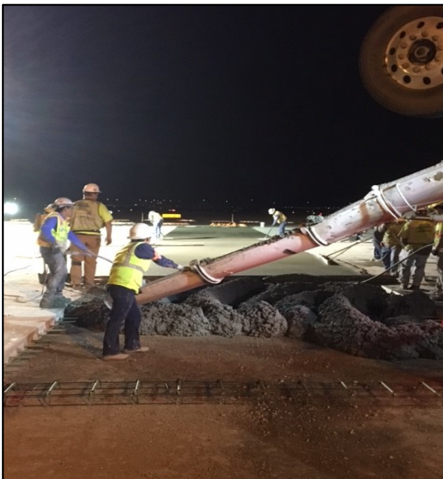
Concrete pouring for North Apron Phase IV
