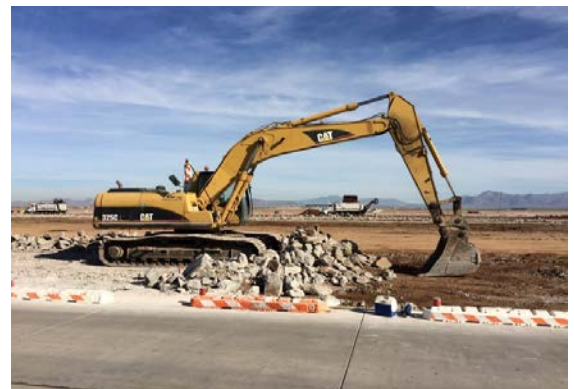
Concrete apron removal
