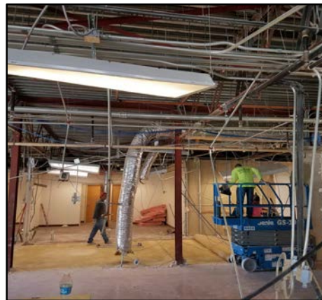
Barrio Brewing Company under construction
