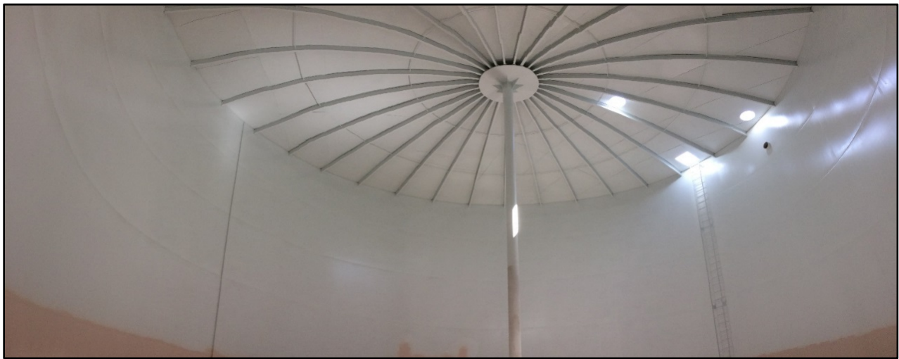
View from inside the recently completed fire suppression tank
