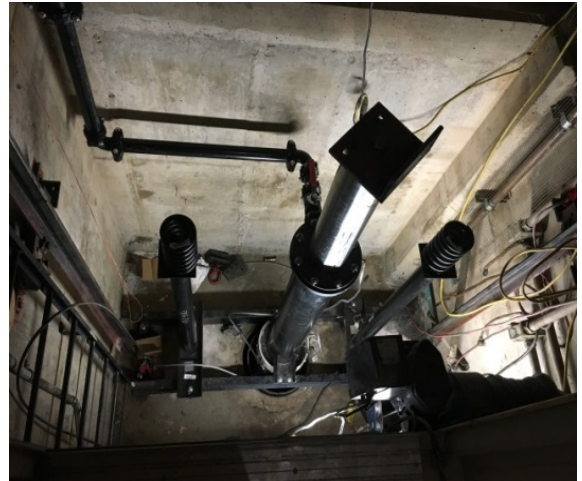
New hydraulic piston in ATCT elevator
