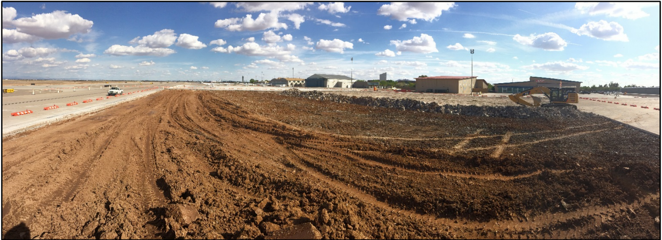
Concrete demolition for Phase IV
