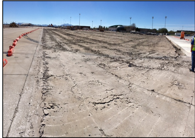
Phase III underway
