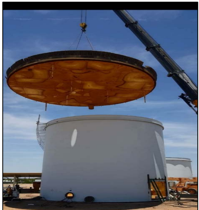
Fire protection system tank roof replacement
