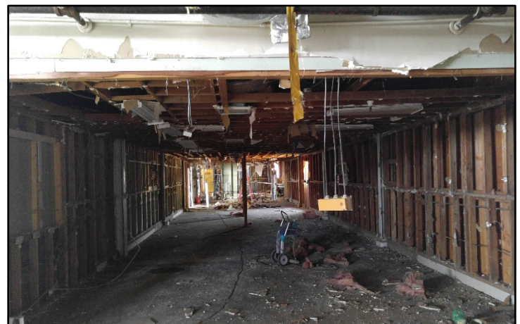
Hangar 32 Construction in Progress
