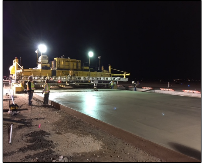
Paving the North Apron Area
