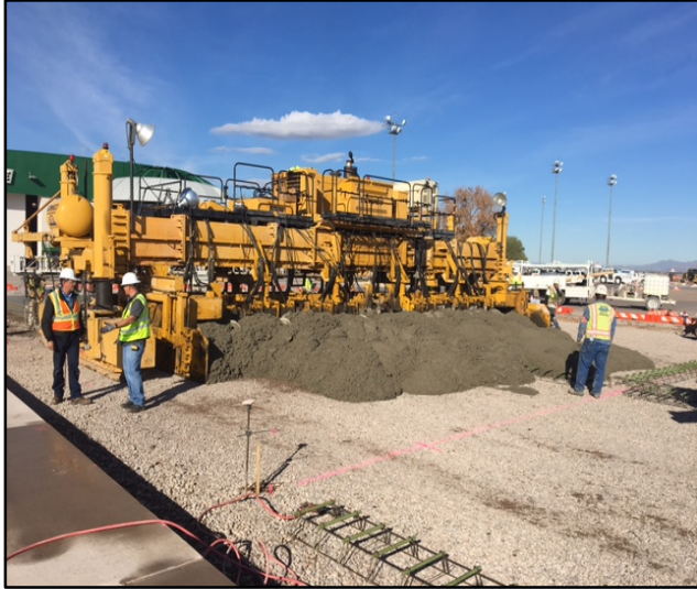
Prepping the North Apron Area
