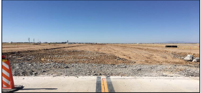
Taxiway Alpha Reconstruction
