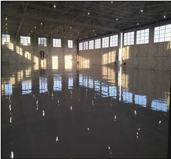
Hangar 32 Aircraft Bay
