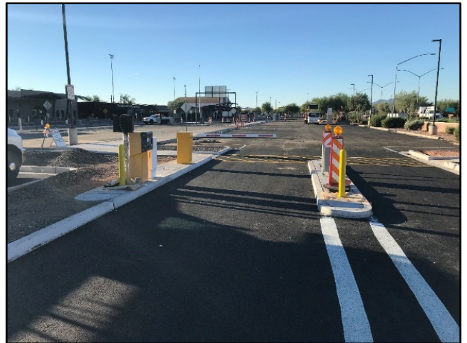
New Hourly Parking Lot Entry Under Construction
