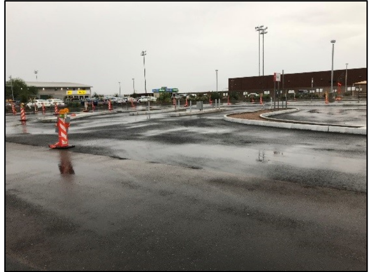
Terminal Roadway Improvement Project
