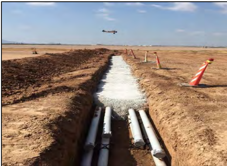
Conduit laid for the final section of Taxiway Charlie
