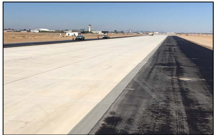
Taxiway Alpha Construction
