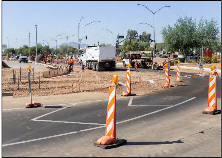
Terminal Roadway Construction Project
