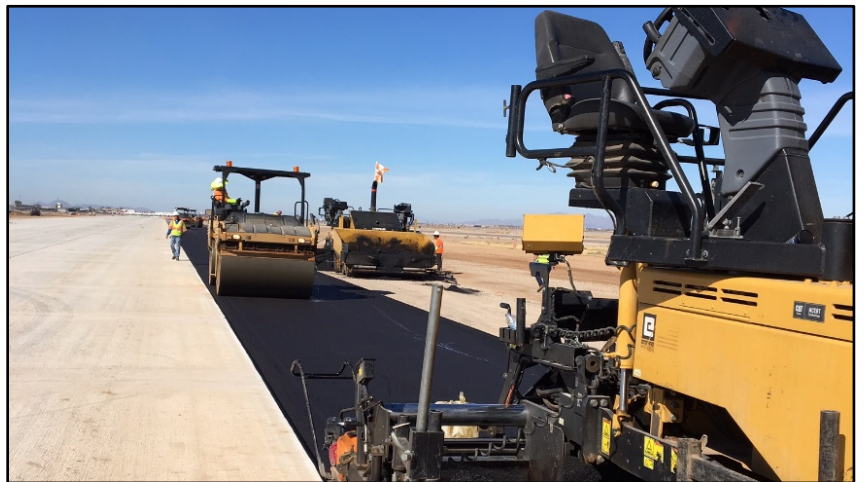
Taxiway Alpha Construction
