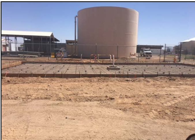
New Operations Wash Rack Under Construction
