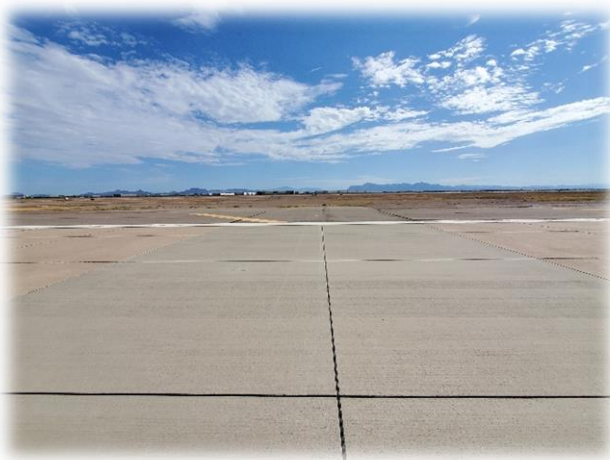
Photo 15 – Storm Drain Trench Crossing RW '12R-30L'
