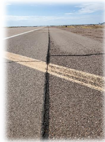
Photo 11 – Existing RW shoulder Pavement Paving Lane Looking South
