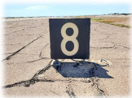
Photo 21 – Existing Distance Remaining Sign
