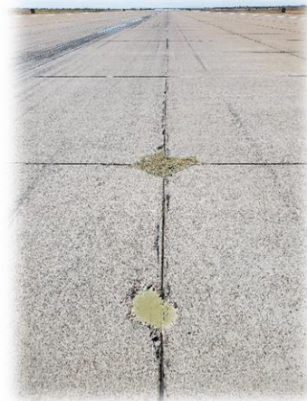
Photo 12 – RW '12R-30L' Concrete Patching
