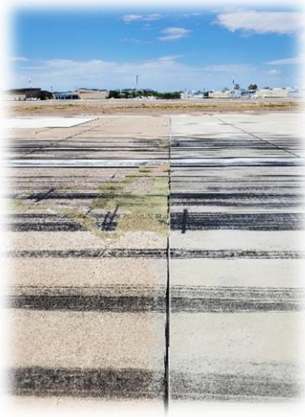
Photo 19 – End of RW '12R' Threshold Reconstruction
