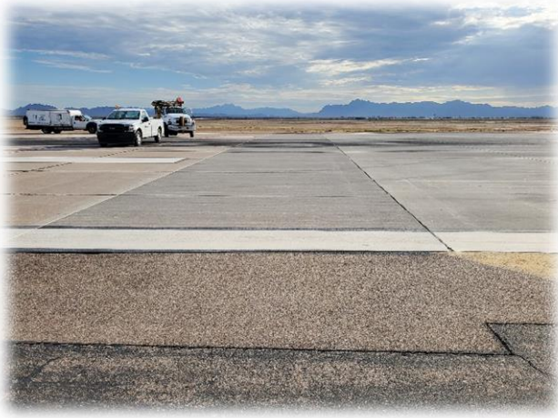
Photo 1 – End of RW '30L' Threshold Reconstruction
