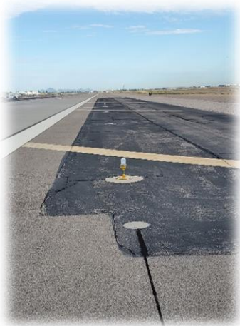
Photo 3 – RW Shoulder Pavement North of TW 'L' (East Side of RW)
