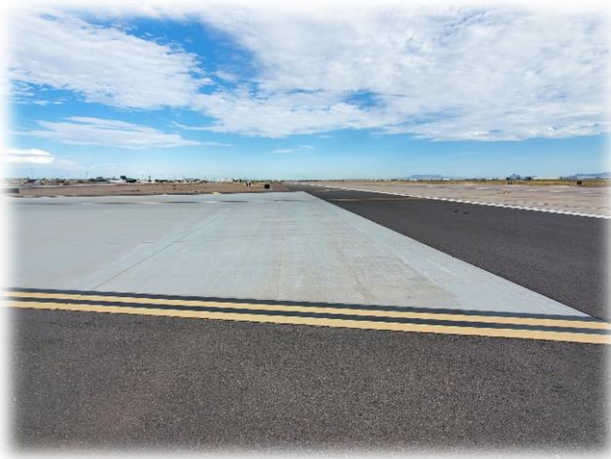
Photo 8 – TW 'K' Intersection with RW '12R-30L' (West Side)
