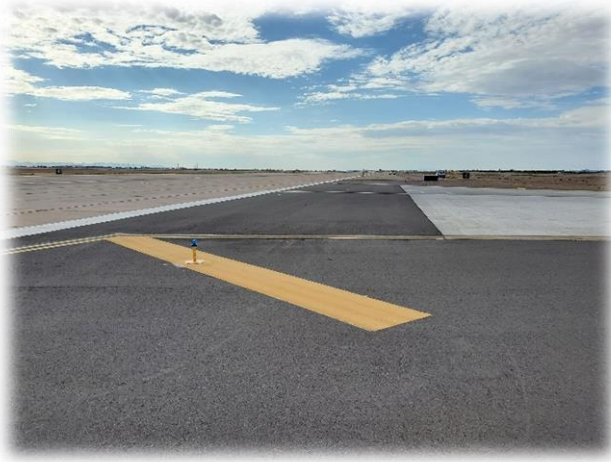
Photo 7 – TW 'B3' Intersection with RW '12R-30L'
