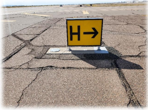
Photo 13 – Existing TW 'H' Intersection with RW '12R-30L'
