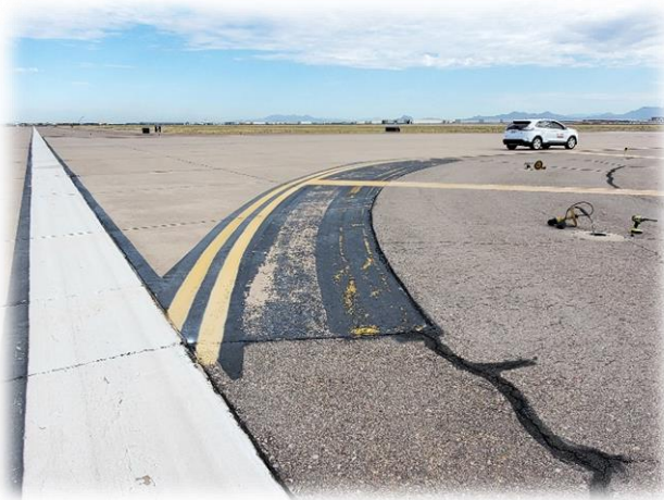
Photo 9 – TW 'K' Intersection with RW '12R-30L' (East Side)
