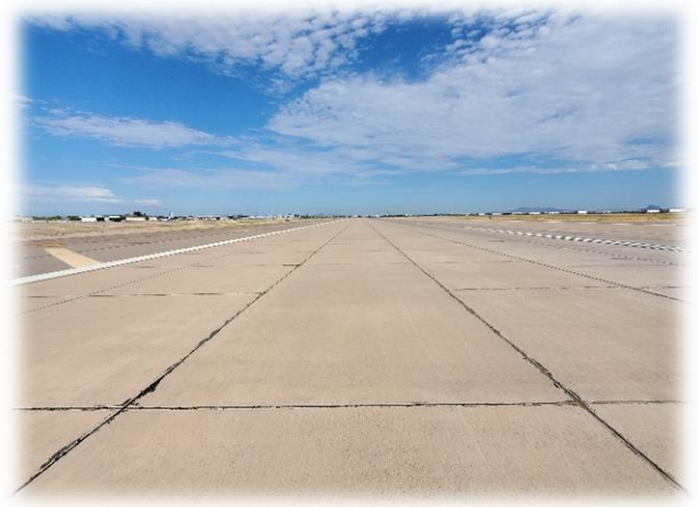
Photo 10 – RW '12R-30L' Looking North
