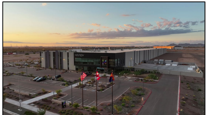
XNRGY's New U.S. Headquarters
