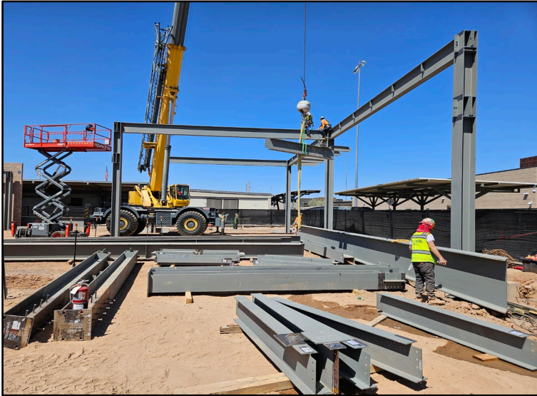
New TSA EDS Facility Under Construction
