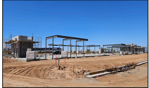
Steel Frame Going Up for SpringHill Suites Hotel
