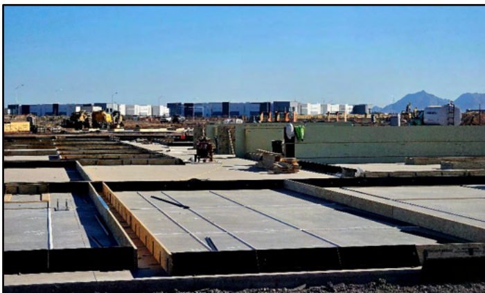
Wall Fabrication for Gateway Commerce Center III
