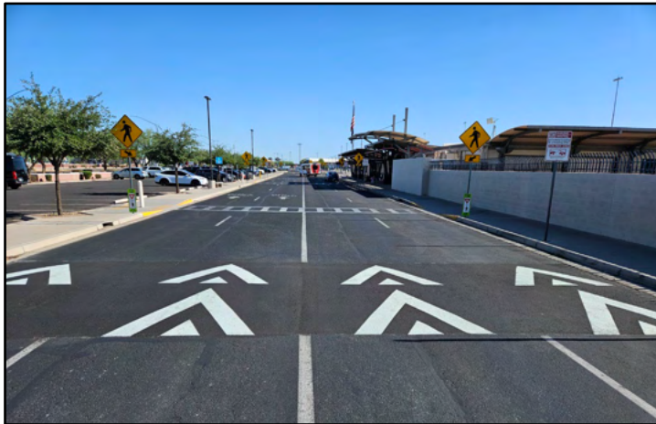
Recently Installed Speed Bump at Gateway Airport
