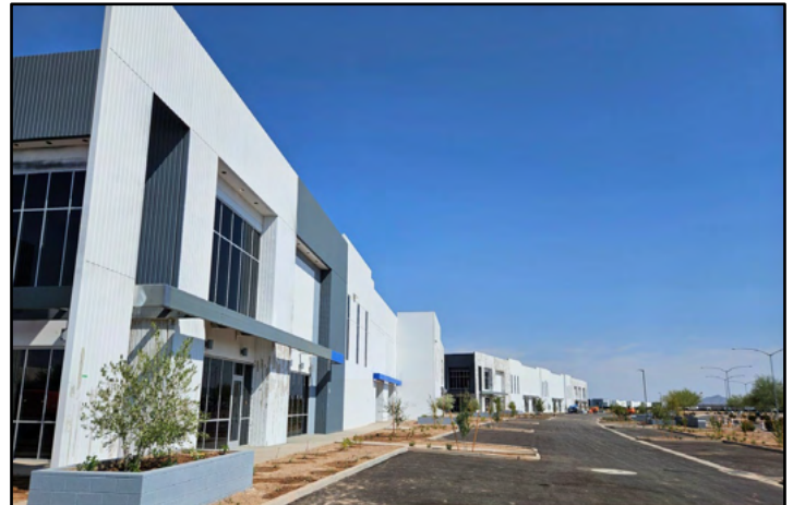
Gateway Commerce Center III Buildings
