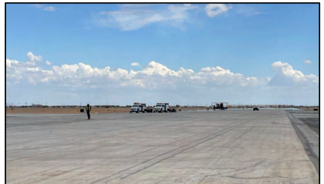
Workers Inspect New Concrete on Runway 12R-30L
