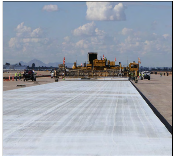
Concrete Being Placed on Runway 12R/30L
