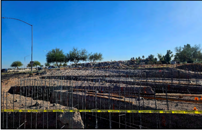
Footings and Framing for New Entrance Sign
