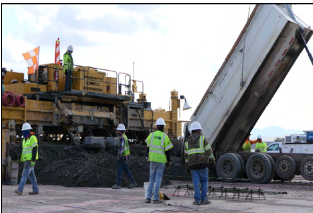
Concrete Being Placed on Runway 12R/30L
